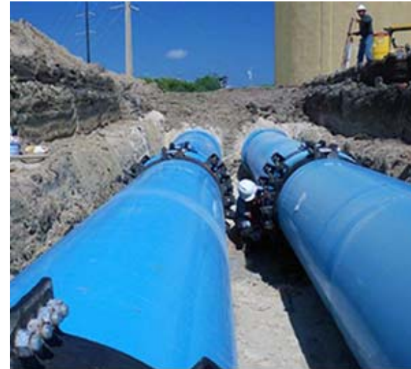
36-inch PVC pipes installed at treatment plant
