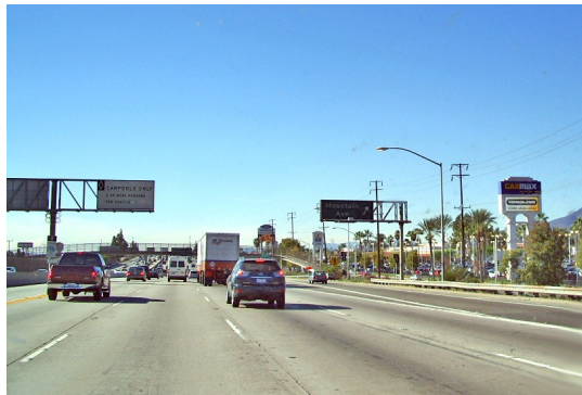
Cluttered highway signage is unsightly and distracts the driver from the road.
