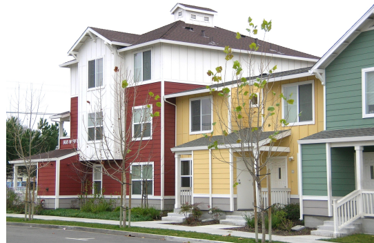
Variable roof forms and height create architectural interest and help larger buildings appear as a series of smaller modules.
