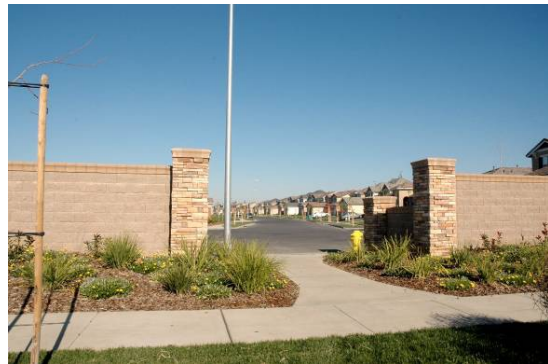
Desirable: Providing breaks in perimeter walls for pedestrian and bicycle access.
