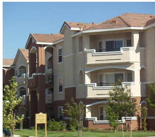
Building design includes projections, articulations, window trim, and recesses that provide design detail and shadow.
